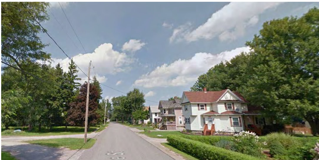
Residential Development in Byron Center
