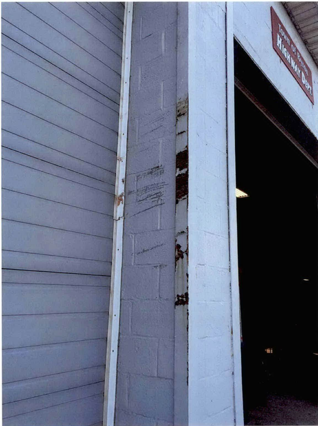
Overhead door jamb, showing effects of inadequate width for trucks.
